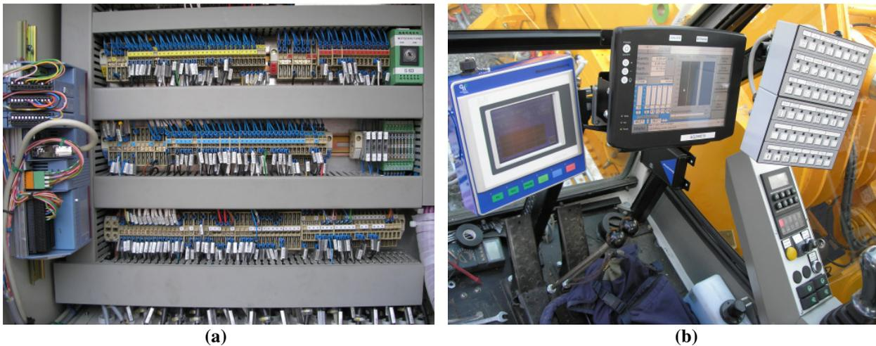
**Figure 2.** Main Control Unit including (a) motherboard (vertical on photo on left) and signal conditioning and (b) real-time viewing and control panels in Operator's cabin
